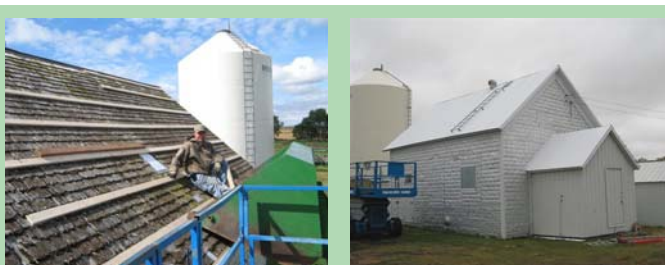
Roger Gutschmidt measured the center point of building’s purlins, then stacked 24 steel sheets with the ends flush and marked where to put in screws. Then he drilled through all 24 sheets at the same time so that all the screw holes were alike on all sheets.
