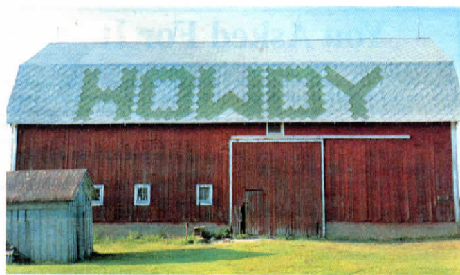
Rentschler plots each design shingle by shingle on paper before starting the job.
