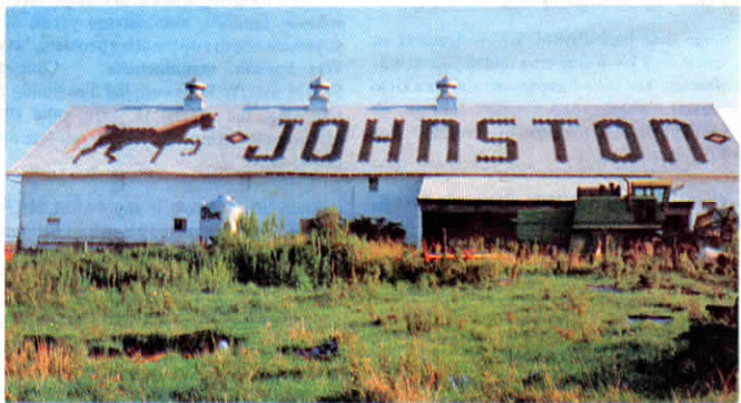
Any design or message can be worked out in shingles on roof.
