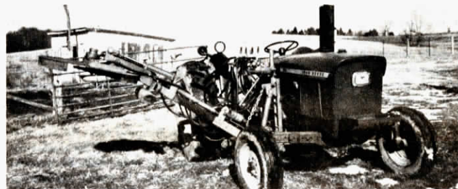
The 3-ft. dia. trimming head, which is adjustable to the desired angle, is mounted on 6-ft. long control arm which also is adjustable for height. Trimming head's distance from tractor is also adjustable "on the go".
