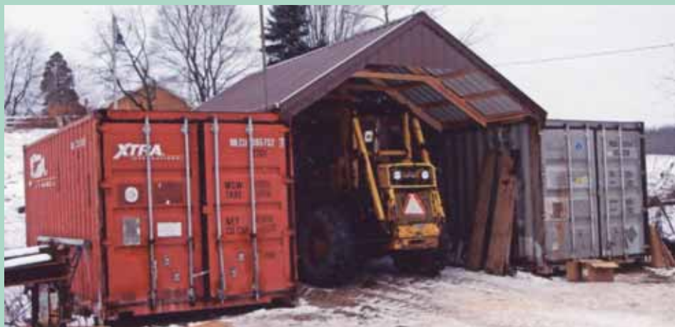
To make a cheap storage building, Butch Soehnlen bought 2 shipping containers, parked them about 20 ft. apart, and built a roof over the space between them.
