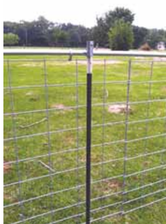
Wire cattle panels hang from top rail that’s held in place by short pieces of pipe on T-posts.
