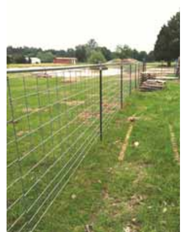
Wire cattle panels hang from top rail that’s held in place by short pieces of pipe on T-posts.
