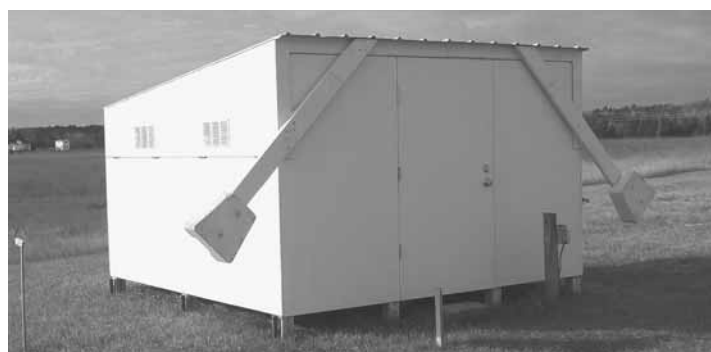
Nick Reed's 9-ft. sq. star-gazing shed is built with a retractable roof. Roof sections are counterweighted and open easily on hinges.
