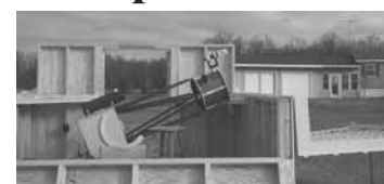
The part of the floor where the telescope sits is isolated from the rest of the floor to eliminate vibration.
