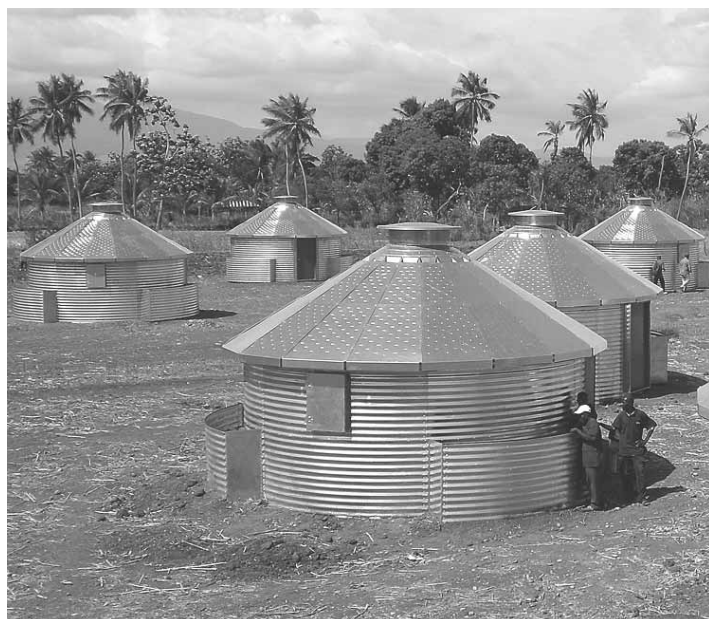
Safe T Homes are modified grain bins turned into mini homes. They're being built for Haitians left homeless after a devastating earthquake in 2010.
