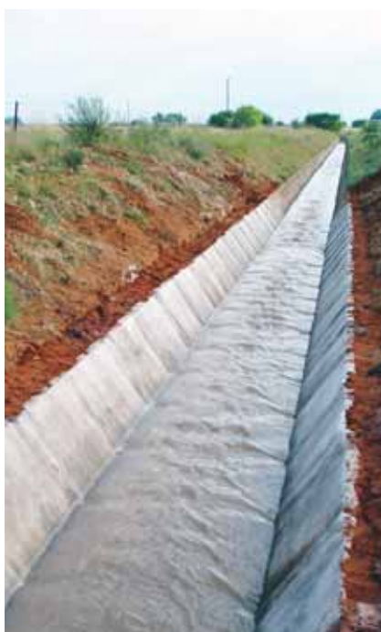
Concrete cloth can be used to create a lined irrigation canal (left). Pre-packaged shelters that use the product are available in the U.K. To construct, canvas is inflated with a large fan and then sprayed with water.
