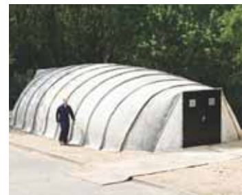
Concrete cloth can be used to create a lined irrigation canal (left). Pre-packaged shelters that use the product are available in the U.K. To construct, canvas is inflated with a large fan and then sprayed with water.
