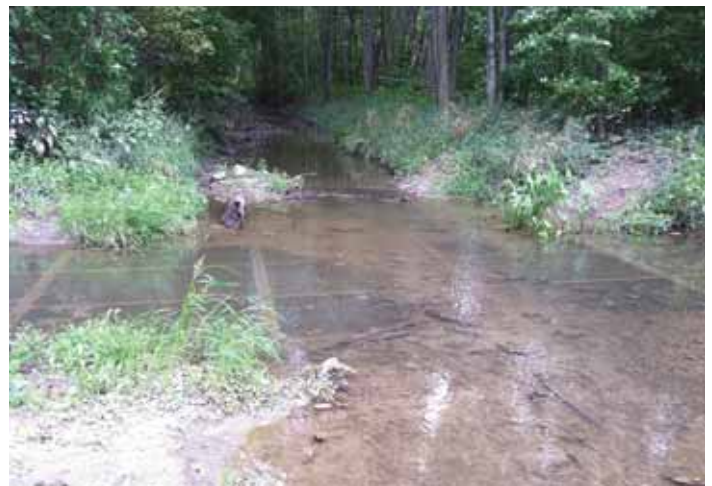
Shallow, concrete well sets across width of stream and is designed to trap sediments that wash off nearby fields. A front-end loader scoops out the collected sediment.
