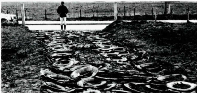
Whidborne uses cut-up tires beads to fill in roadways.
