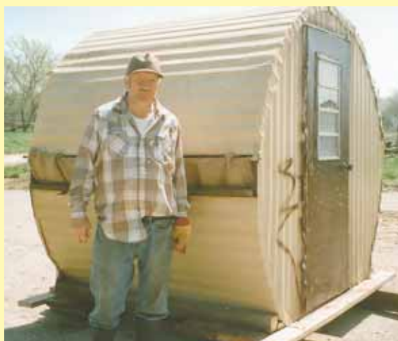
Jim Rogers made this skid-mounted hunting blind by wrapping metal siding around big bale feeder rings sitting on their sides.
