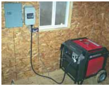
Load-sensing control switch starts a gas-powered generator automatically whenever it senses a demand for power.
