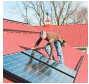
Building specs were upgraded to accommodate the solar panels' extra weight.
