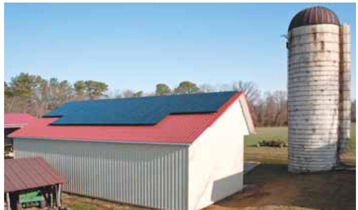
Michael and Eugenia Wootton installed 42 solar panels on a new metal building to cover most of their electricity needs. They figure it'll have a 5 to 7-year payback.
