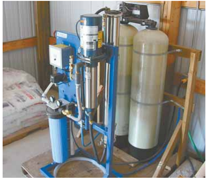
Farm-size water treatment system can produce about 400 gal. of mineral-free and neutral pH water per hour.
