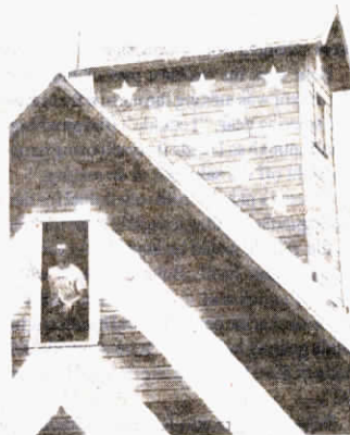
The main part of the barn is in red and white stripes while the coupola is painted with stars on a blue background.
