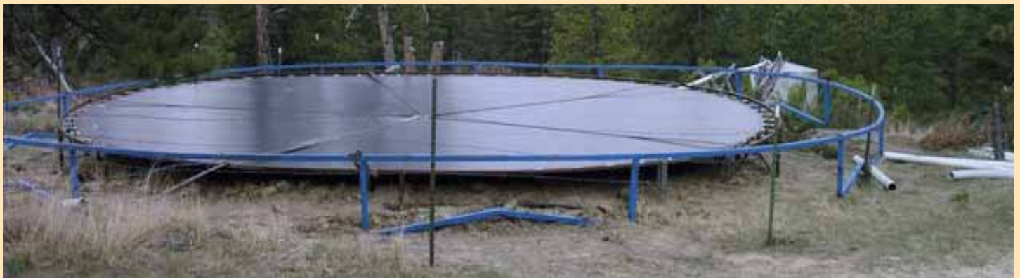
Giant poly “trampoline” catches rainfall in remote pastures and funnels it to a center drain for storage.
