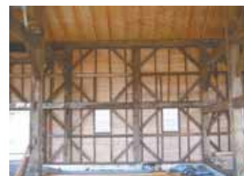
Barn is fitted with big doors to bring in equipment to work on.
