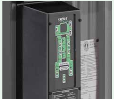
The FireStar II controller controls the outdoor wood furnace and can store data and communicate with other devices.
