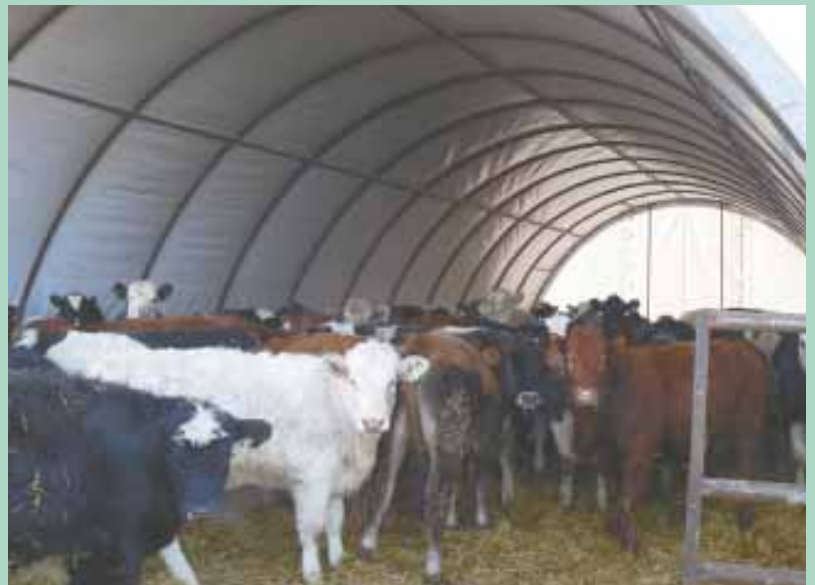
Silver Stream also makes a line of free-standing shelters that don’t require sidewalls. They’re available with either single steel hoops, as shown here, or steel truss hoops.
