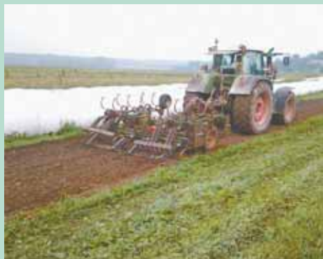
At an 800-cow dairy in Pennsylvania, Perma-Zyme was used to treat a farm lane used daily to haul manure. The owner applied the product himself, diking it into the surface. He says the lane is now very solid and he plans to use Perma-Zyme on other troublesome farm paths next spring.
