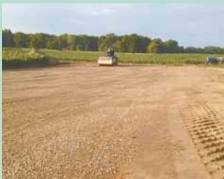
This solid silage pad was created at a cattle farm in Virginia. The area had always been a wet trouble spot.
