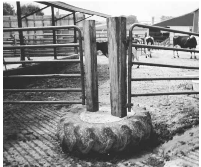
Swinging gates hang on posts anchored in concrete-filled tractor tires. The Huneke's use the portable posts to divide a large pen on their dairy farm.
