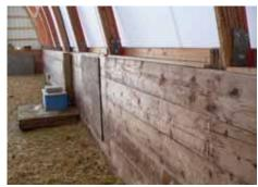
Wood hoop barns are available in 30, 36, 38, 40, 42 and 44-ft. widths, built to any length. Can be easily finished with end walls and doors.
