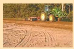
Farm equipment is all that is needed to prepare the soil and mix the solution. An industrial roller or packer will do the best job compacting. Discs and roto-tillers may also be used to mix the soil. After the correct grade is achieved, compacting is key.
