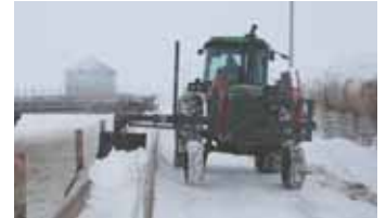
Unit uses a rubber "squeegee" bolted to a 1/2-in. thick steel blade.
