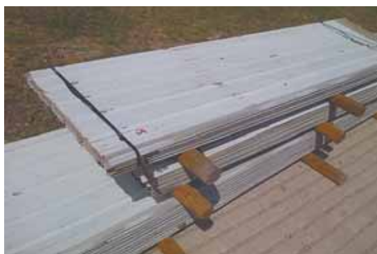
John Taylor tears down old steel buildings, then bundles and sells the used steel to farmers.
