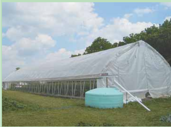
Linda and Randy Naeve equipped their Pro Solar Style High Tunnel with rain gutters on either side. Harvested rain water is used to irrigate plants inside and out.
