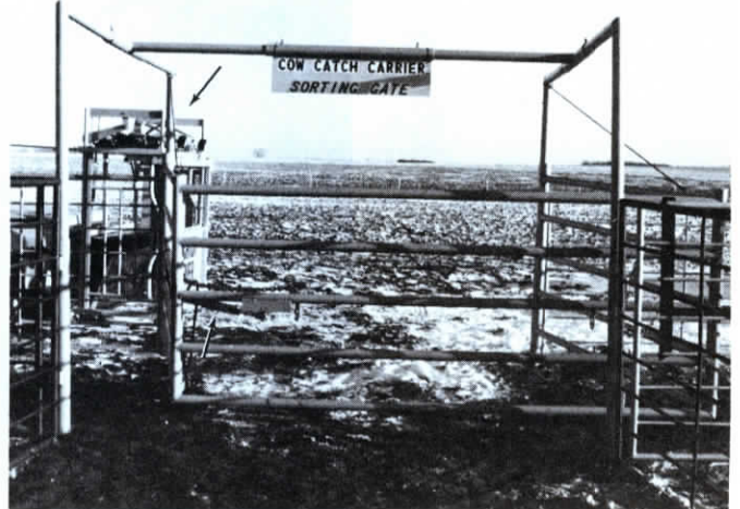
Above installation is only half completed. Main alleyway will be extended, and a companion swinging gate added, so cattle can approach sorting gates from either side, as shown in drawing below.
