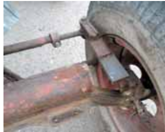
They welded tabs of scrap steel over each other to connect the truck steering knuckles to the tractor's tie rods.
