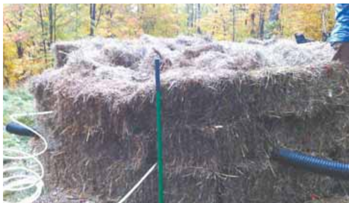
Hay bales provide a sturdy wall to contain compost and heat layered pipe coils. Project shown above was set up to heat a nearby greenhouse.
