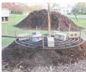
Hay bales provide a sturdy wall to contain compost and heat layered pipe coils. Project shown above was set up to heat a nearby greenhouse.
