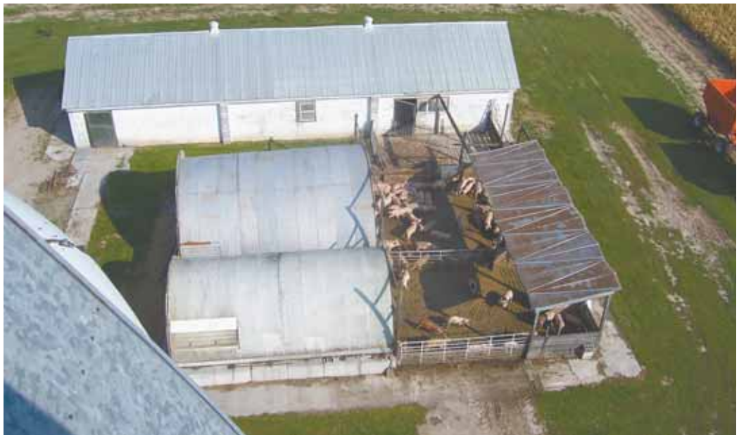
Eric Hartemink converted 2 old grain bins into inexpensive, "quonset-style" hog shelters. He tipped the bins on their side and removed the roofs, then mounted the roofs on metal posts to create a carport-like shelter that covers his feeders.
