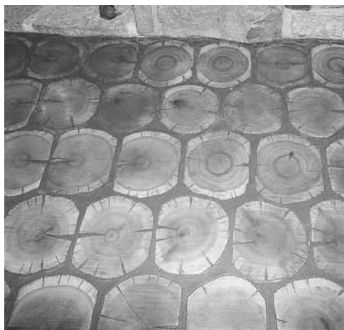
Steve Lee installed this cordwood floor in his Wisconsin home. “It’s a time consuming process to get the wood cut, laid, glued, sanded and varnished. But it turned out pretty neat,” he says. Lee suggests reading Richard Flatau’s book “Cordwood Construction”.
