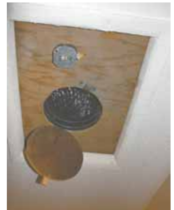
An old furnace blower is connected by flexible ducting to a collar mounted on access door to attic. A light switch on door is used to turn fan on or off.
