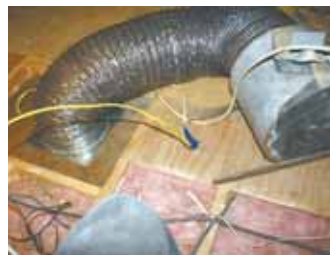
An old furnace blower is connected by flexible ducting to a collar mounted on access door to attic. A light switch on door is used to turn fan on or off.
