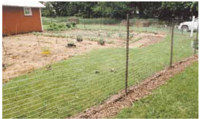
Galvanized chicken wire fence is buried 6 in. deep in ground to keep digging animals out. Mulch keeps weeds down and eliminates the need to get close with a mower.
