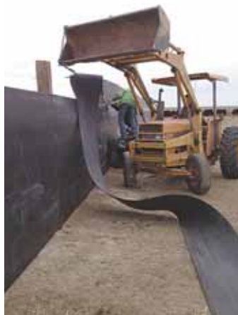
Old conveyor belting was used to build this 8-ft. high windbreak on a ranch.
