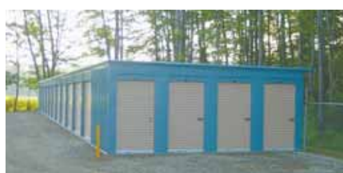
By using prefab parts, Flexospan can custom-engineer a building to whatever size and configuration the customer wants. The partitioning system makes it easy to change the size of units.
