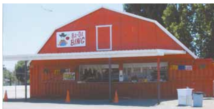
From the front, Jim Aira's fruit and vegetable stand looks like a shiny red barn. It's actually a used shipping container with a false barn front built over the top.
