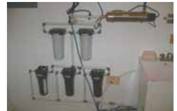
Treatment includes pumping water through three .5-micron filters, then two .2-micron filters and finally a UV sterilizer.
