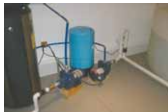
Treatment includes pumping water through three .5-micron filters, then two .2-micron filters and finally a UV sterilizer.
