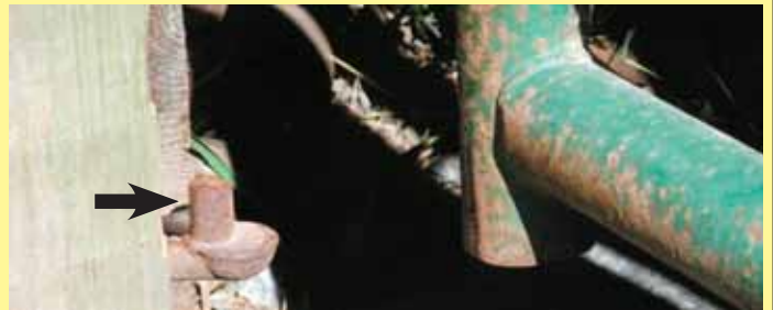
Burns sets end of gate onto cut-off gate hinge.
