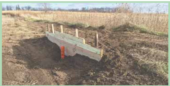
To keep heavy rains from washing out his field waterways, Lorn Manthey installed 6-ft. high wooden fences behind his tile standpipes and in front of soil berms.
