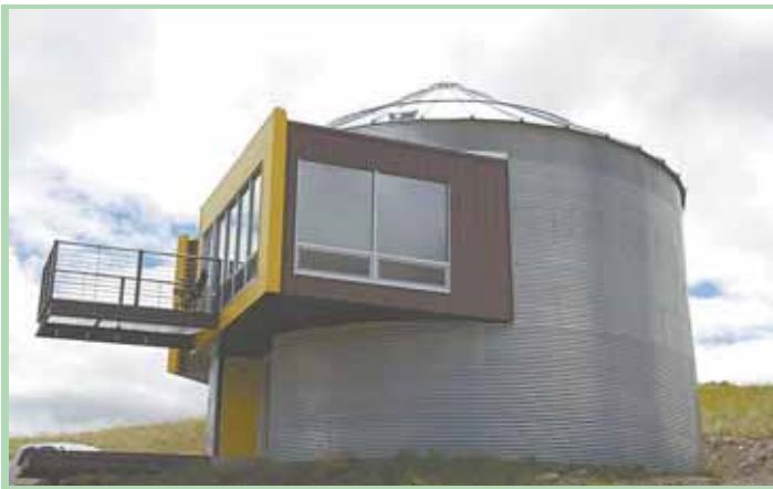
Two-story grain bin home has “bump outs” painted bright gold/yellow to match the original MFS logo still on the corrugated bin. A 7-ft. steel deck with bar grate flooring is just outside the living room.
