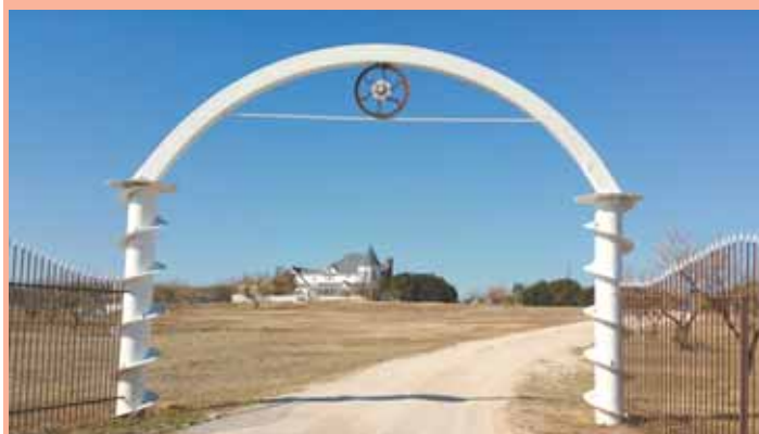
A pair of 30-ft. augers set in concrete footings mark the entry to Kent Irons' driveway, honoring the family's history of custom combining.
