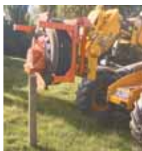
Loader-mounted "vibrator" drives posts into ground.
