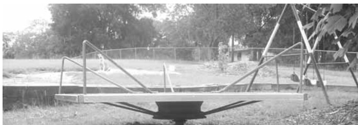
Wagner framed out a steel deck and then pop-riveted 1/8-in. thick aluminum onto it.
