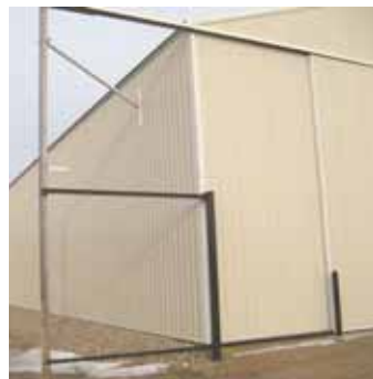
On windy days, the 20-ft. sq. doors on Gutschmidt's machine shed would catch wind like a big sail. The sliding door supports he designed keep that from happening.
