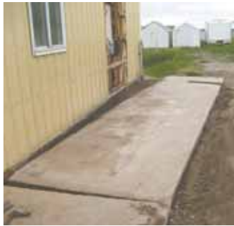
Roger Gutschmidt used a big tractor to tow this 25 by 6-ft., 5-in. thick concrete slab to a new location. He cut a hole in the slab, then tunneled under it with a long air nozzle to blast out dirt. Then he slipped a log chain through the hole and pulled the slab away.
