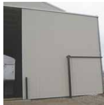
On windy days, the 20-ft. sq. doors on Gutschmidt's machine shed would catch wind like a big sail. The sliding door supports he designed keep that from happening.
