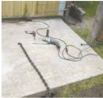
Roger Gutschmidt used a big tractor to tow this 25 by 6-ft., 5-in. thick concrete slab to a new location. He cut a hole in the slab, then tunneled under it with a long air nozzle to blast out dirt. Then he slipped a log chain through the hole and pulled the slab away.
