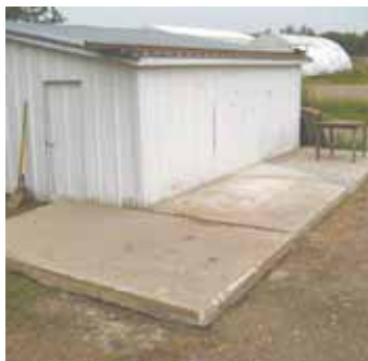
As Gutschmidt headed uphill over some uneven ground, the slab broke into 2 big pieces. He pulled them one at a time to the new location and set them in place. He then filled the big crack between them with concrete.
