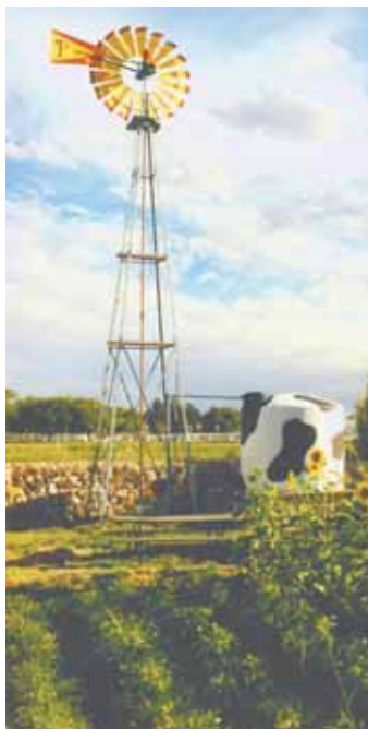
Robert Peterson brought this 33-ft. tall windmill home in pieces in back of his pickup, then put it up by hand with no crane or other lift needed. He rigged up a gin pole at top of tower.
