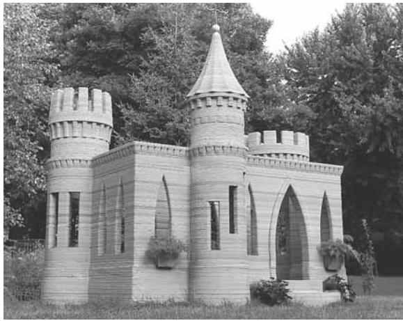
Engineer Andrey Rudenko "printed" out this authentic looking castle layer by layer, using a machine he built himself. Castle measures 15 ft. wide, 12 ft. deep and 9 ft. tall.
