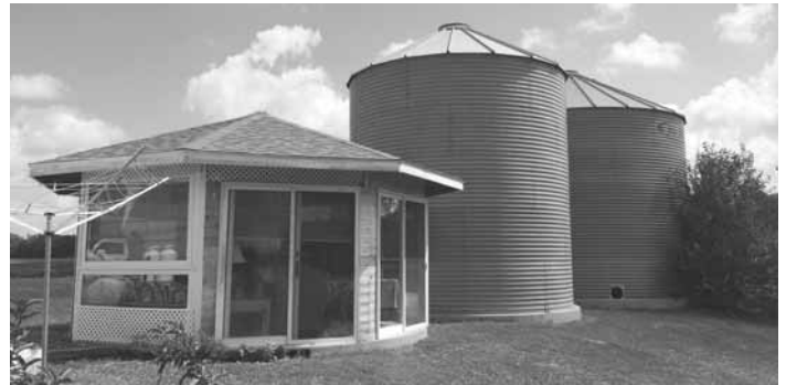
Ruth Macias had a local contractor build this 6-sided, screened-in gazebo and anchor it to the concrete slab from an old grain bin.
