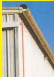
Rain Gutter Made From Irrigation Pipe (Page 3)
