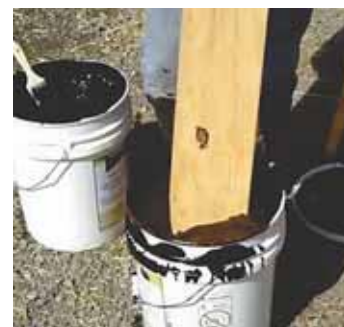
RubberizeIt works great to coat the bottom of fence posts to protect the wood from rotting.
