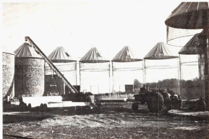
Kleptz fills his 10 semi-circled corn cribs with one 50-ft. elevator.
