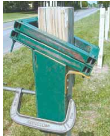
Cut-off template is bolted to a couple of short, angled 2 by 4's and a piece of plywood that connects them. Entire assembly is held on post with a C-clamp.
