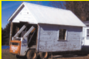
Skid Loader Takes Shed For A Ride (Page 19)
